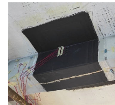
Manufacturing Patch Process to repair the composite structure
