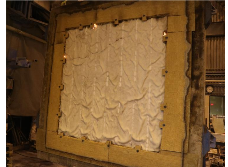
Fire exposed side after test
